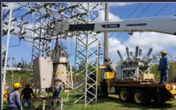
34.5 KV Breaker Upgrades
